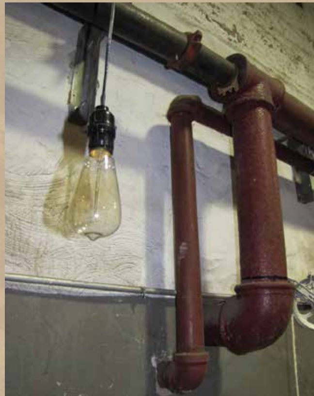
Christine Altman, Pock-ET installation in progress Photo credit: Leslie Kaufman
