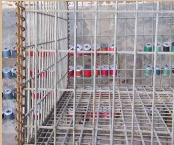
Pam Bowman, Seamless Installation in progress
